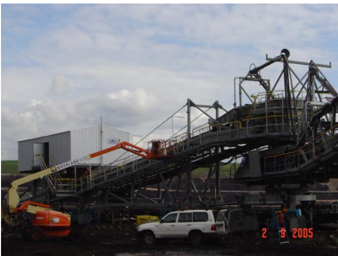
Site assembly of TS2 Stacker
