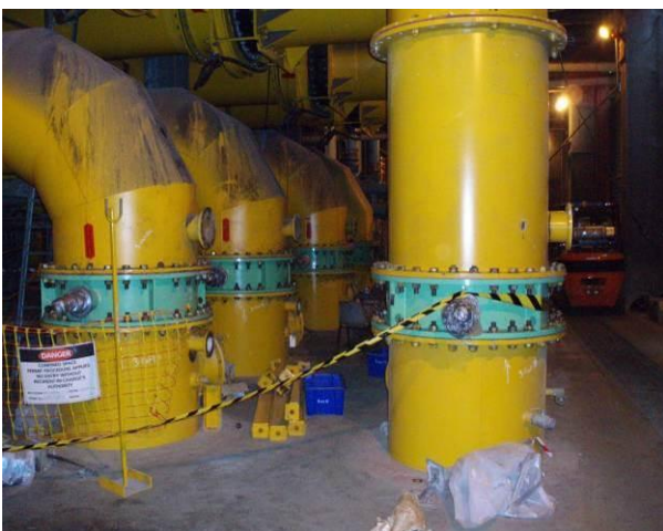
Condenser valve replacement
