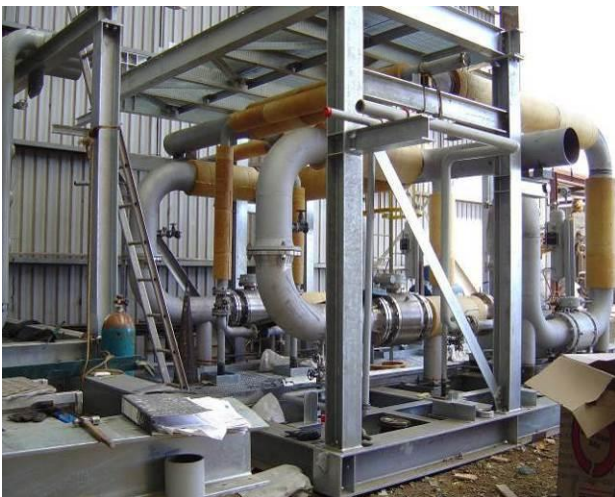
Bass Gas Pipe rack insulation
