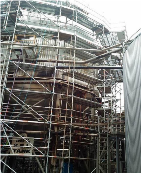
SBL Tank Top Strake Replacement
