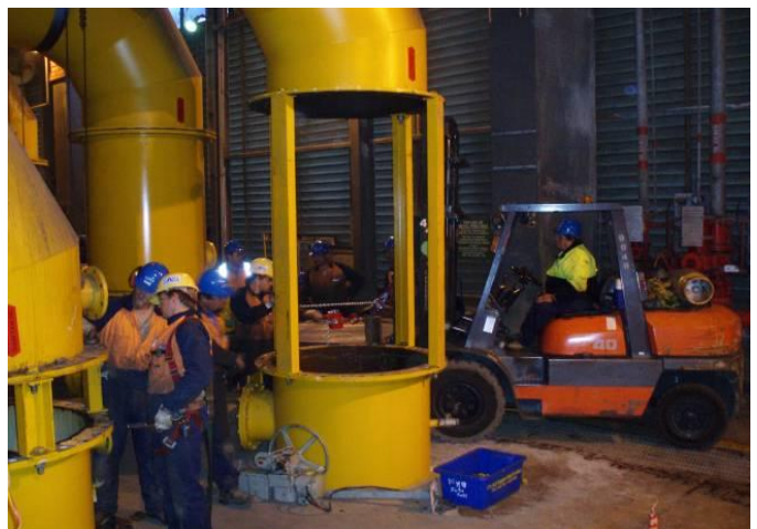
Safe removal of Condenser conduits
